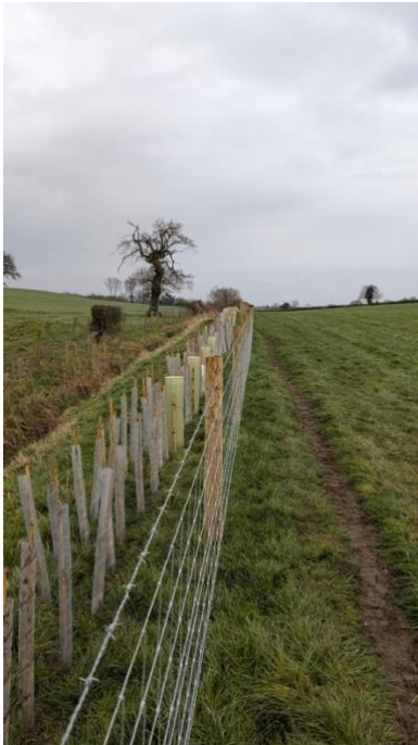
New hedging and fence, Hill House Farm, 2025
