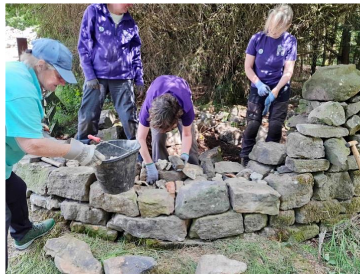
Above: Repairing drystone walls
