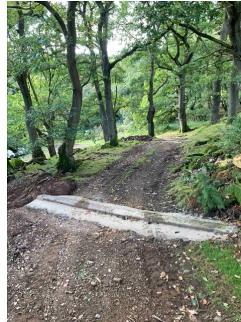
A cross drain at Skell Gill, 2022
