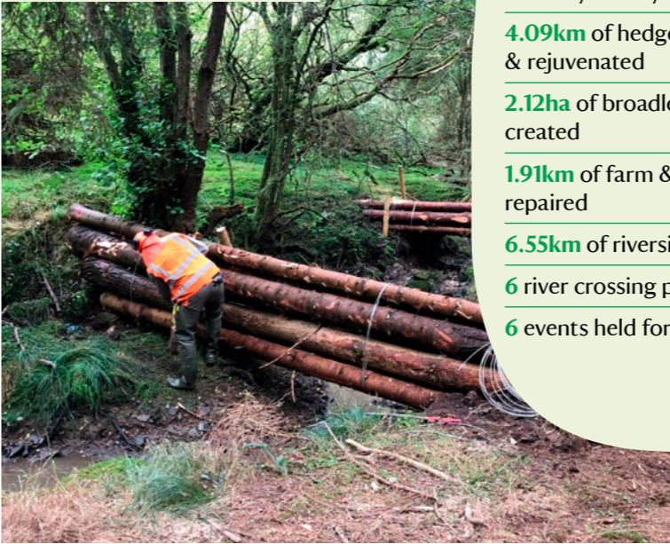
Leaky dams installed on a tributary of the River Skell
